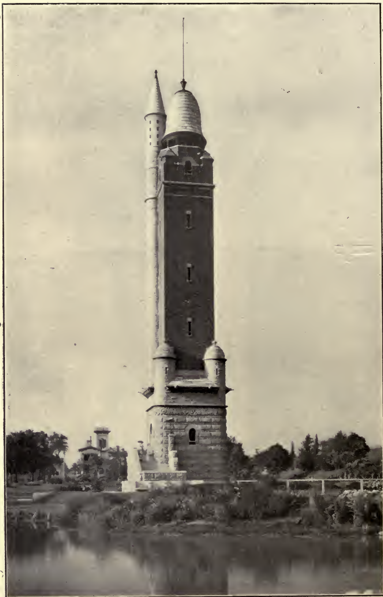
FIG. 61.—ST. LOUIS WATER-TOWER.
